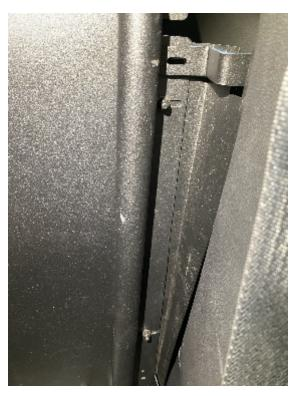
11. Install center extension to partition using 1/4 acorn nuts and washers (Fig 8.)
